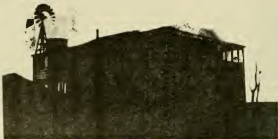
2. An exterior view of the same bunk house shown above.
